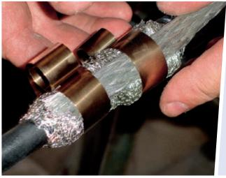
The earth wire is cut to 1.5 times the length of the removed section of the outer protective coating, and pulled over the neighbouring protective tube in such a way that approximately 100 mm are left bare and free at both ends of the earth strand.
