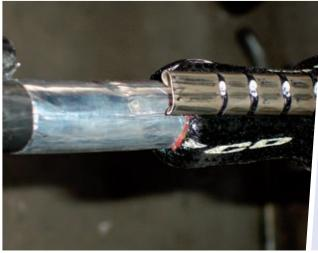
It should be easy to recognise that the green dots on the seal have almost completely disappeared. Glue will leach slightly out of the sleeve end lying on the flame-retardant foil. The white indicator line under the sealing edge is clearly visible.
