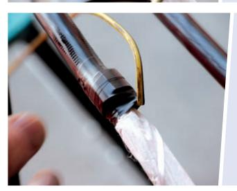
Then the V-clip and laminated sheath are wrapped with three layers of plastic tape. The drain wire can be cut off or additionally wrapped around the clip. If necessary please note any supplied customer instructions for this.
