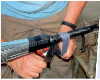
The outer sheath is cleaned until it is oilfree, roughened across the cable axis and then heated with a low flame to hand-hot temperature.
