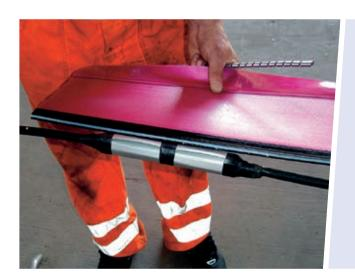
Line up centrally the seal for the heatshrinkable sleeve. It must extend beyond the protective padding by the same length on each side.
