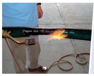
When shrinking the sleeve, begin in the middle. For this procedure heat the complete area of the sleeve and shrink it towards one end.
