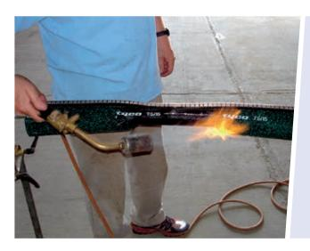
When shrinking the sleeve, begin in the middle. For this procedure heat the complete area of the sleeve and shrink it towards one end. Then work on the other end.
