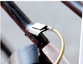
The V-clip of the shield continuity wire is laid sideways around the edge of the cut fold of cable and closed tightly with combination pliers.
