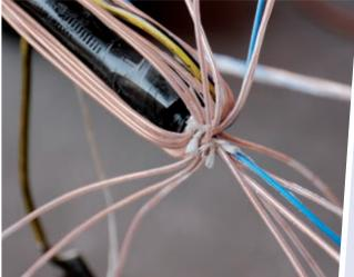
When splicing the copper cores the correct stranding order must be observed.
