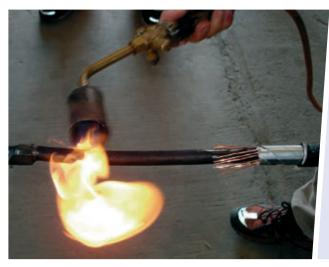
Following this the cleaned and roughened areas are heated with a burner until they are hand-hot.
