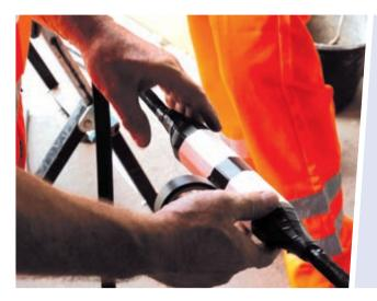
The lamellar areas of the protective padding should be unwound with adhesive tape.
