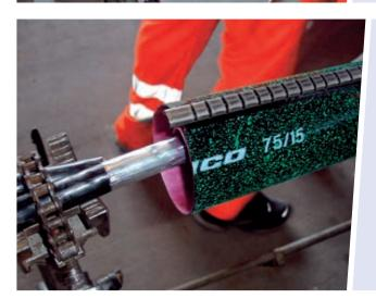
Before shrinkage the sleeve should be centred. The two flame-retardant foils which reach slightly into the sleeve on both sides may serve as orientation.
