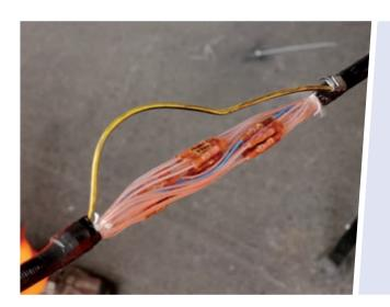
Staggered splices result in a narrow joint.
