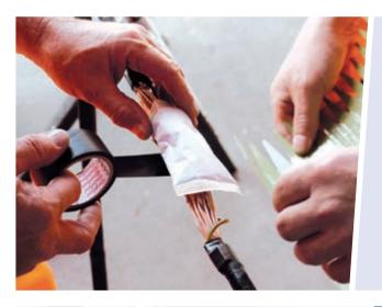
Before installation of the actual heatshrinkable sleeve, the drying agents supplied with the packaging should be fixed around the core splice with adhesive tape.
