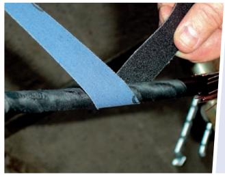
Once the oil has been removed the laminated sheath is roughened across the cable axis with an emery cloth. Any pitted areas in the sheath must also be roughened.
