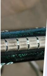
The shrinking process is over when the seal has evenly shrunk, the green colour pigment in the sleeve material has disappeared and the white indicator line is easily visible under the sealing edge. At the ends small amounts of glue must be seeping out of the cable.
