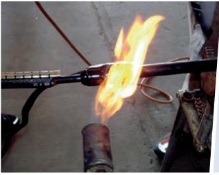
The protective wrap is heated with a low flame until the tape shrinks and glue seeps out at the overlaps.
