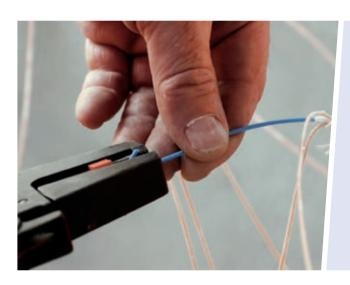
The cores are individually stripped of insulation with the help of a suitable cable stripper.
