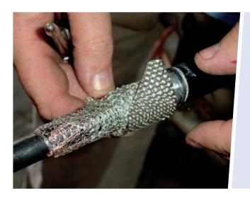
The supplied contact plates are preformed according to instructions, laid around the copper fabric tape and wrapped and secured with one layer of the copper fabric tape (with a max. 5 mm overlap).
