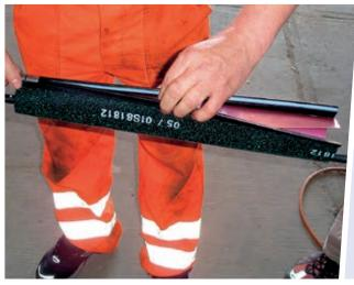
The seal is laid completely around the splice and the sealing edge pulled up.
