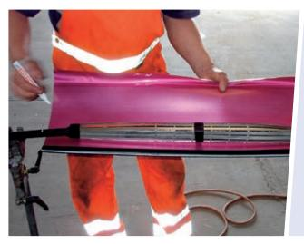
The wrapping on the conical ends of the metal protective padding should be clearly visible. The seal for the heatshrinkable sleeve is laid centrally over the connecting point and the projectionmarked on at least one side of the laminated sheath.
