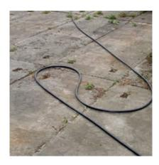
If the cable is to be laid out in sections this may only occur in so-called 'figures of eight' (picture above), which are set out according to the cable diameter (note the bending radius!). Torsion of the cable can then no longer occur.
