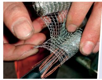
The copper fabric tape should be wound according to instructions in a single layer around the armouring and shielding wires.
