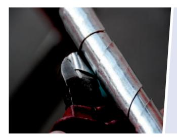
The upper layer of steel band is sawn into and can now be carefully unwound using a pair of pliers.
