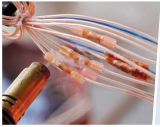
After installation the crimp splices are carefully shrunk with a burner. Released glue and the closely fitting plastic protect the bare copper joint mechanically and against dampness.
