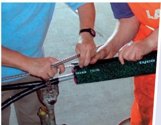
The heat-shrinkable sleeve is placed centrally around the metal protective padding and closed on both sides with the sealing edges. The connection clip is placed between both ends of the sealing edges in the centre of the sleeve.
