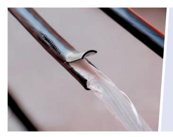
An incision is made in the remaining laminated sheath in two places at a maximum distance of 15 mm apart, each cut being 30 mm long.
