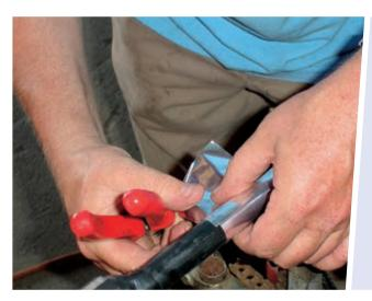
The flame-retardant foil (self-adhesive aluminium foil) is attached so that it is laid over the marked line approximately 10 mm towards the inner sleeve. In this way it reaches a maximum of 10 mm into the sleeve, whilst the greater part of the foil remains outside the heat-shrinkable sleeve. The foil should be smoothed over with a blunt tool, for example the smooth handle of a pair of pliers or the handle of a hammer.
